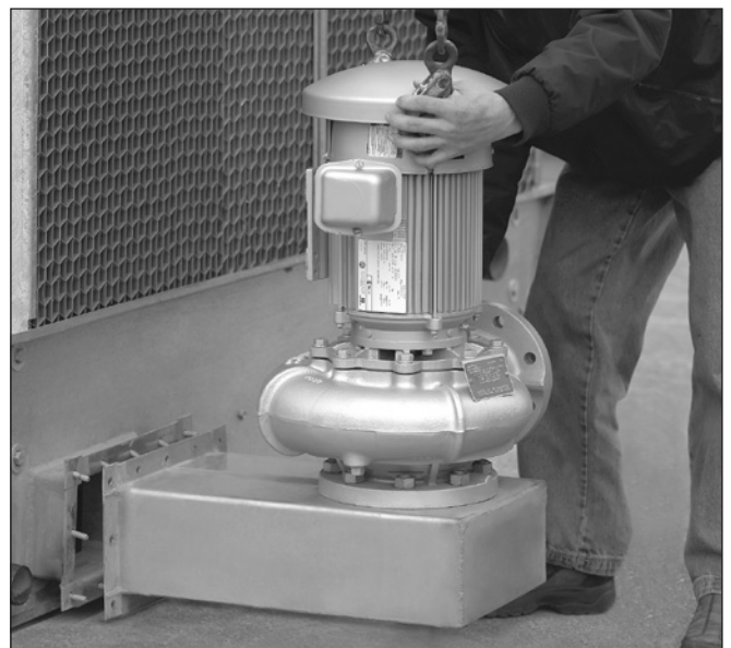
Figure 20 – Detachable pump base assembly
