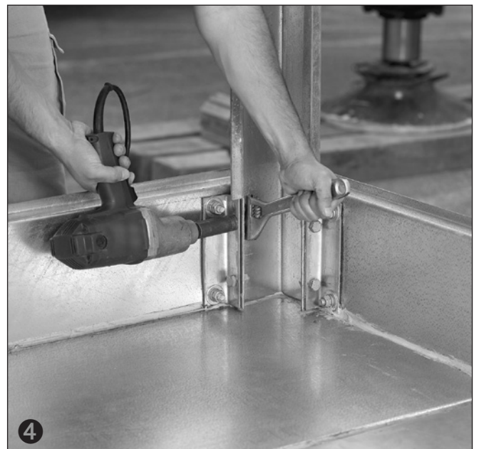
Step #4: Tighten all hardware
