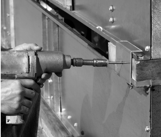
Figure 7 – Removal of shipping channels
