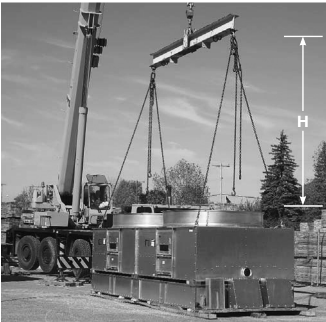
Figure 5 – Lifting arrangement for fan section
