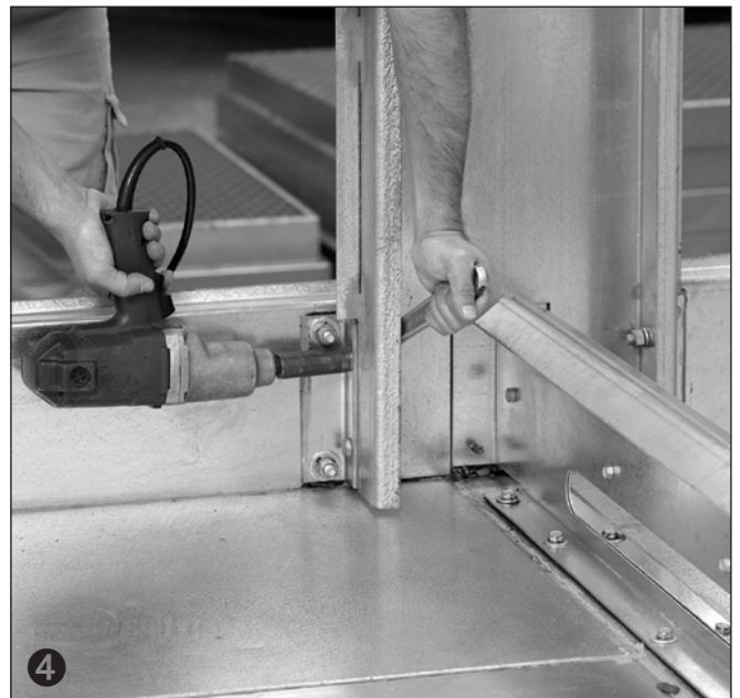
Step #2: Install vertical support and tighten hardware
