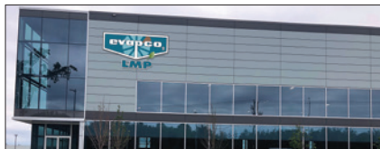
EVAPCO LMP, Laval, Quebec
