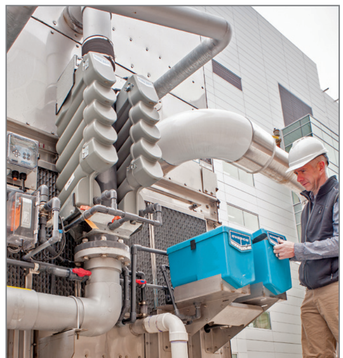
Smart Shield® Factory-Mounted Water Treatment System
