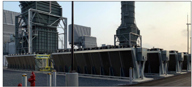
eco-Air Air Cooled Heat Exchangers Factory Assembled Packaged Units Located at Grade
