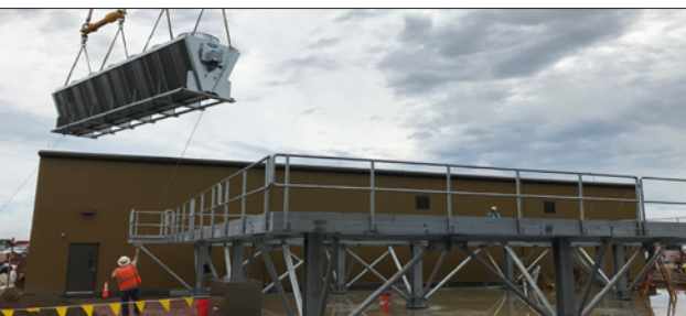
eco-Air Air Cooled Heat Exchangers Easy Installation of Factory Assembled Packaged Units
