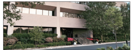
EVAPCO Dry Cooling, Bridgewater, New Jersey
