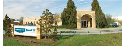
EVAPCO Alcoil, York, Pennsylvania
