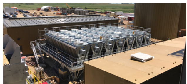
eco-Air Air Cooled Heat Exchangers - Factory Assembled Packaged Units Installed on Common Structure
