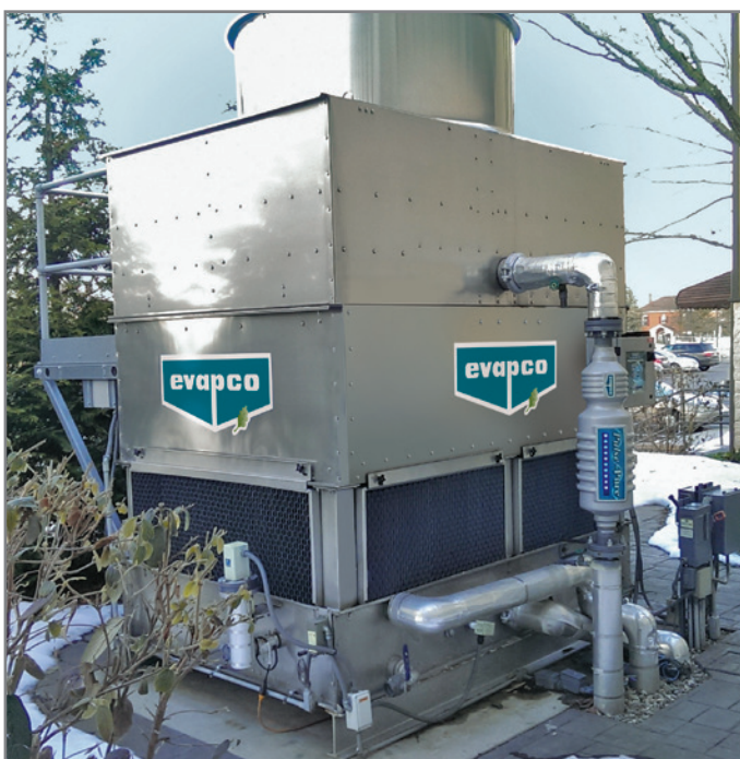
AT Cooling Tower with optional Pulse~Pure® non-chemical water treatment system
