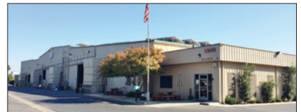
EVAPCO West, Madera, California
