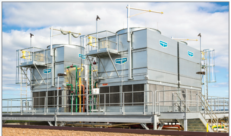
ATC-E Evaporative Condensers with optional external service platform
