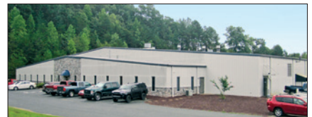
Tower Components, Inc., Ramseur, North Carolina
