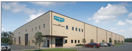
EVAPCO Key Building, Taneytown, Maryland
