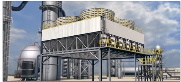
Advanced Technology ACHE Saves Plot Plan, Aux. Power, and Lowers Noise
