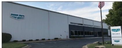
EvapTech, Inc., Edwardsville, Kansas
