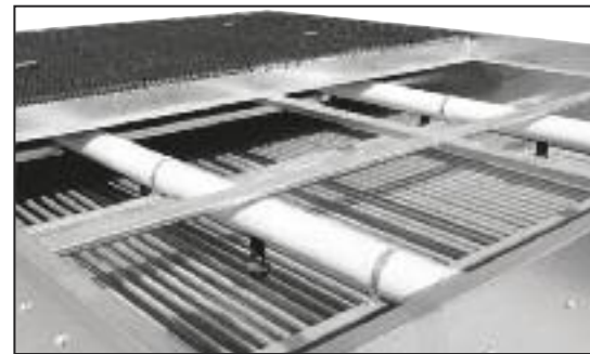
Drift Eliminators Removed for Coil Inspection
