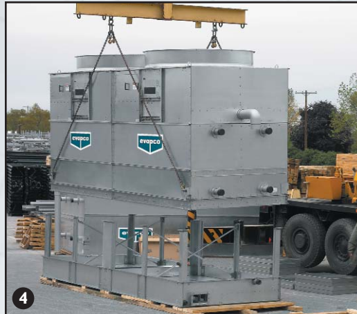
4 Mount Coil/Fan to Basin Section
