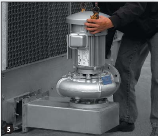
5 Mount Pump and Piping
