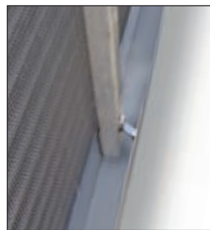
Fully Welded Pan Hanger Brackets
