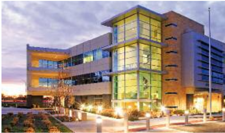
LARGE HVAC APPLICATIONS
