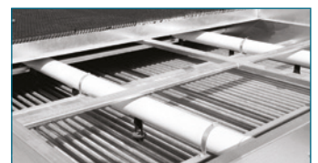
Drift Eliminators Removed for Coil Inspection
