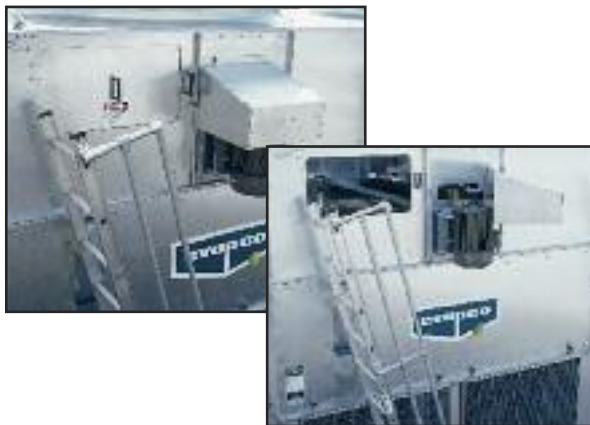
External Motor Mount (with optional ladder)
