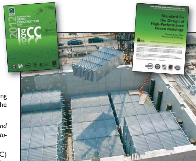
Thermal ice storage meets the demand reduction requirements of the IgCC and ASHRAE Std. 189.1
