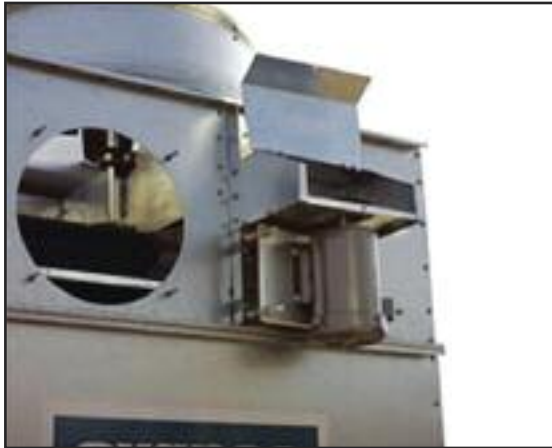
External Motor Mount (with swing away cover)
