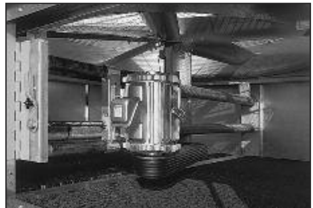
Motor Base Assembly
